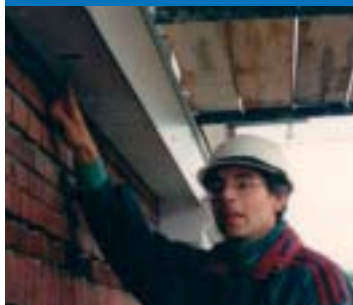
Sluif in gootbekisting
